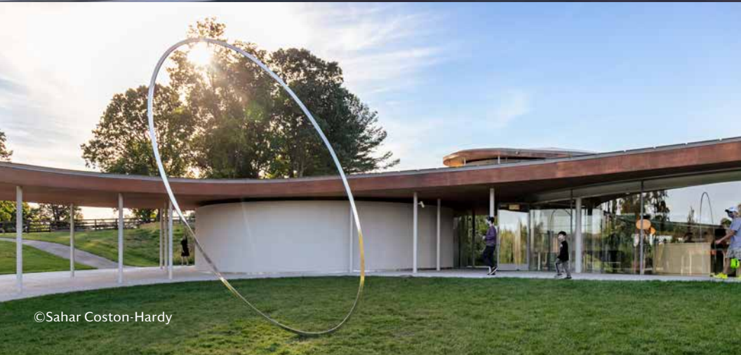
Centerbrook Architects, courtesy: New Canaan Library
